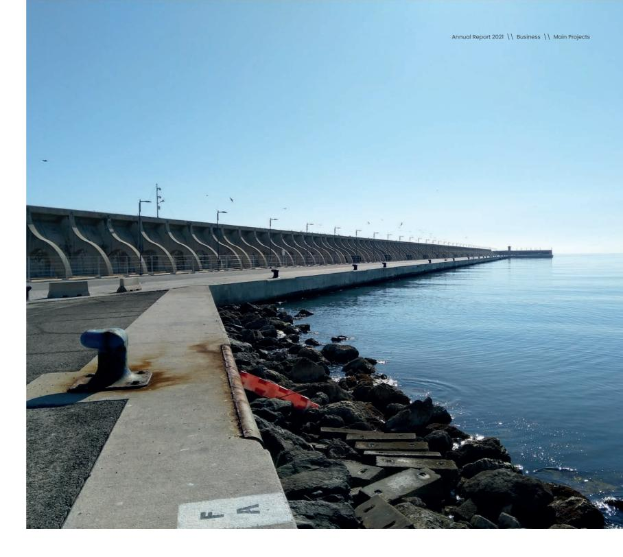
Works to be undertaken include the displacement of existing installations and protection during the works, the chipping of the vertical wall covering and all sides of the buttresses and removal of the existing accessible reinforcement, the demolition of the upper slab and the backfilling with mass concrete of the areas of cover removed, as well as the existing space between and under the buttresses, including the current installations area and previously demolished sidewalk areas.
